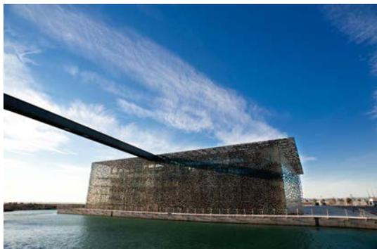
The “Musée des Civilisations de l’Europe et de la Méditerranée” at the Port of Marseille. The building is constructed of a total of 1,100 cubic meters of concrete – in the form of prefabricated concrete slabs – and 250 cubic meters of in-situ concrete. The dark-gray color tone of the airy mesh-like concrete structure was provided by the LANXESS pigments Bayferrox 330 and Bayferrox 318.
